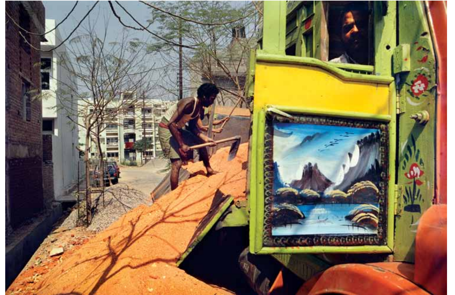
New construction site, South Delhi, 1991
